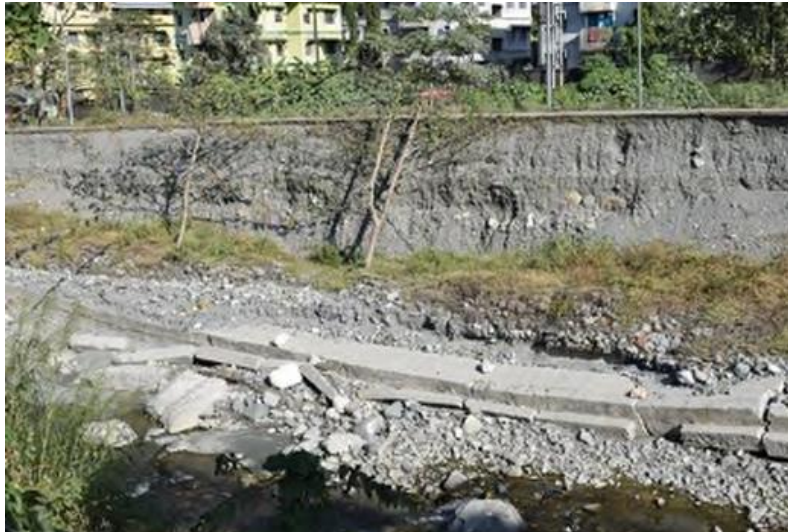
Figure 68: Armor on the banks of the Omchhu have failed in places. Photo taken in 2016.
