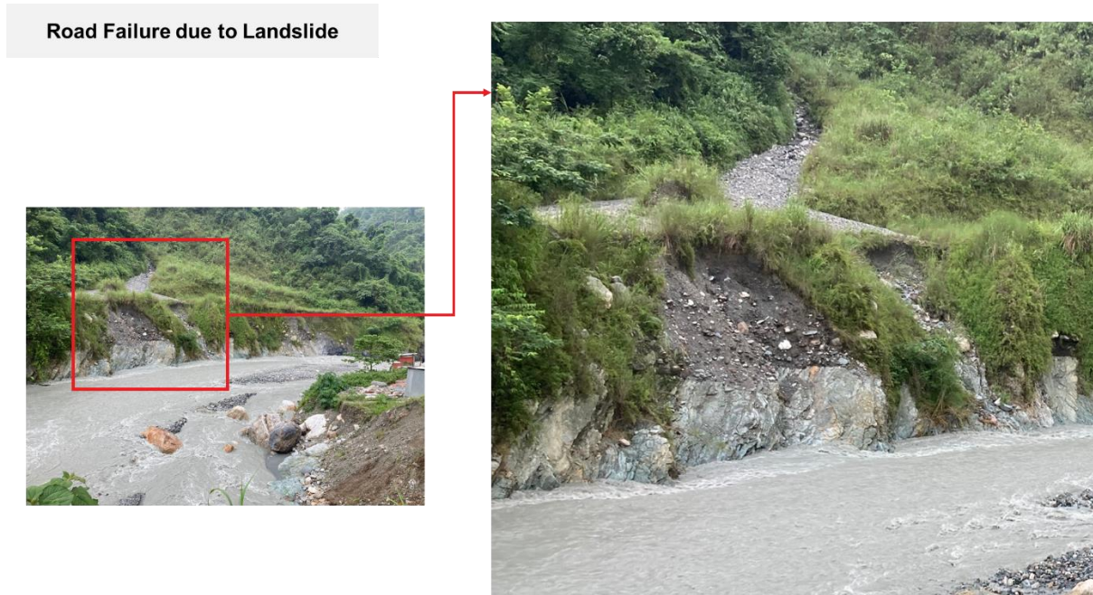
Figure 116: Road failure due to debris from landslide
