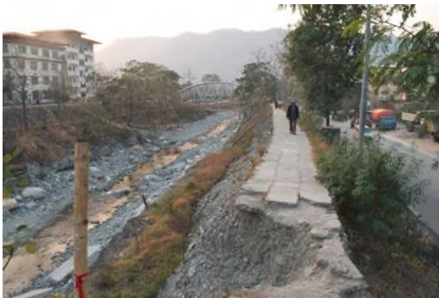
Figure 67: Bunds flank the Omchhu along both banks through Phuentsholing. Note the ground elevation behind the bund is lower than the walking path on top of the bund.
