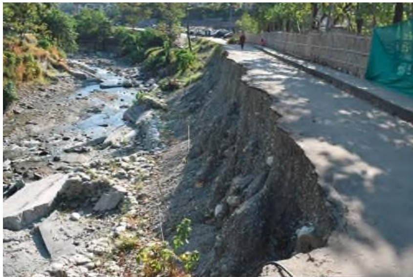
Figure 72: The bund on the left bank of the Omchhu has been narrowed by erosion near the new parking garage. Photo taken in 2016 prior to garage construction.
