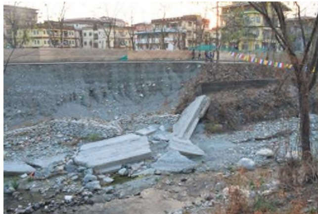
Figure 73: Concrete slabs collapsing into the channel due to undermining of the bank armour could constrict the channel and lead to upstream deposition. Photo taken in 2017.
